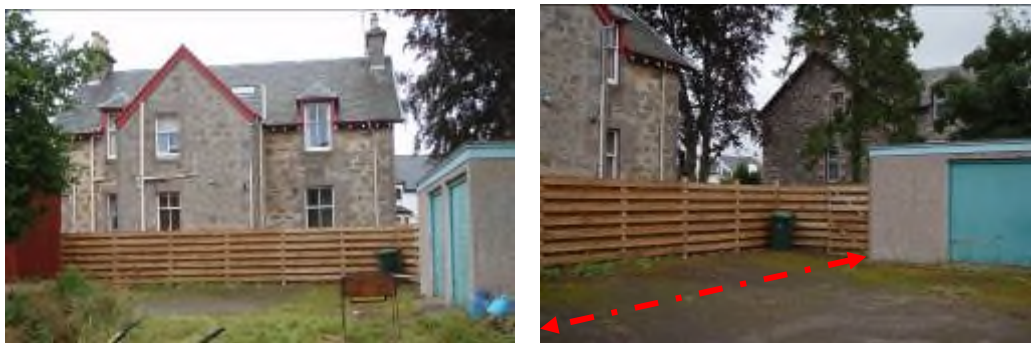
Fig. 10: Existing fence immediately to the rear of the Listed Building. The current proposal would result in a new fence being erected in a revised position in line with the gable end of the garage.
